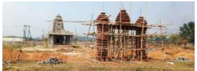
Pondoloi Temple Construction WIP
