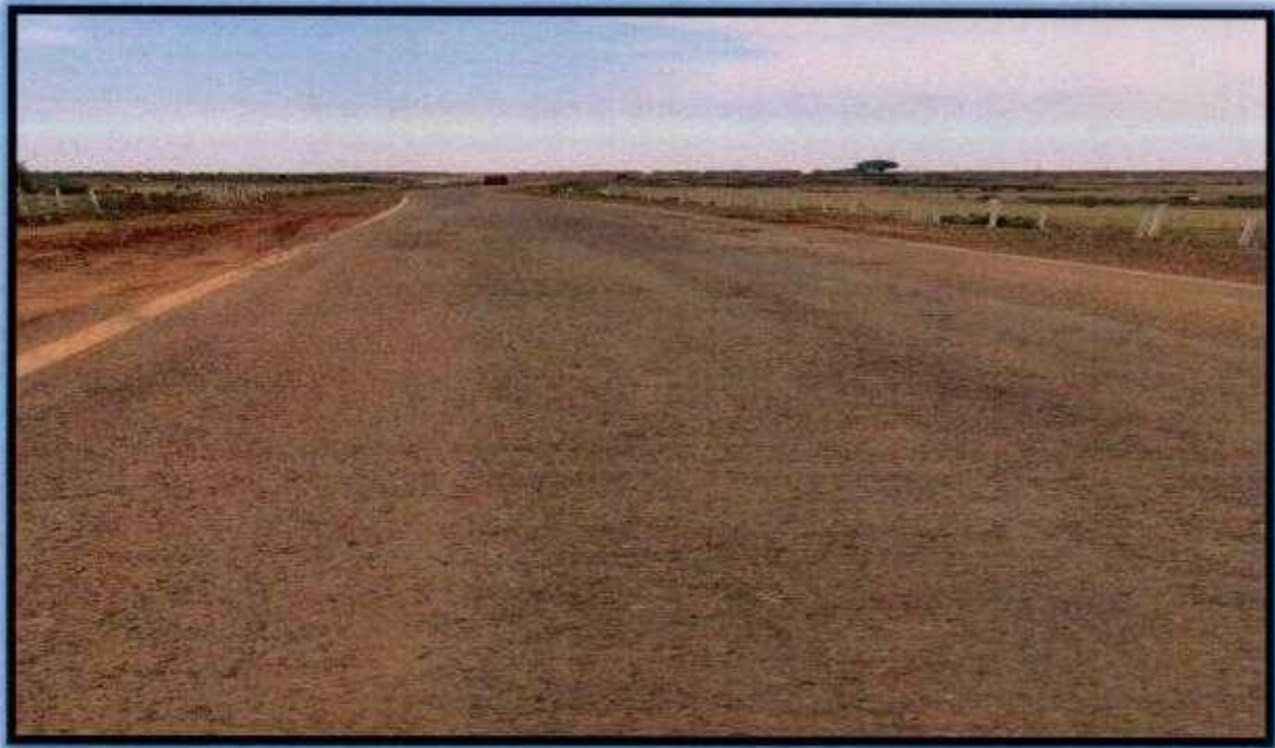
View of Black top road constructed up to pit head to reduce dust problem.
