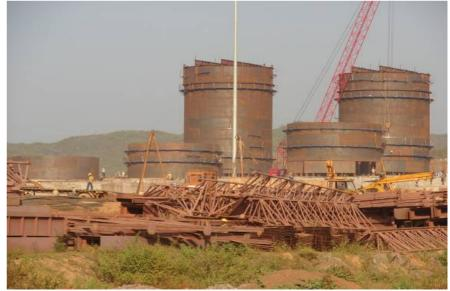
PPTs – 5 tanks shell erection in various stages (TK-202, 23 204, 205,102 & 104)
