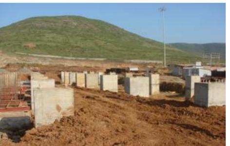
Evaporation Package – Foundations ready for structure columns erection
