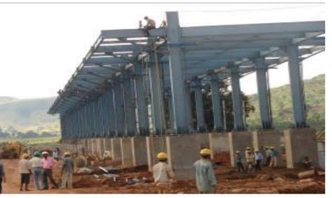
Pipe rack- PR 022, 48 columns & beams erection completed
