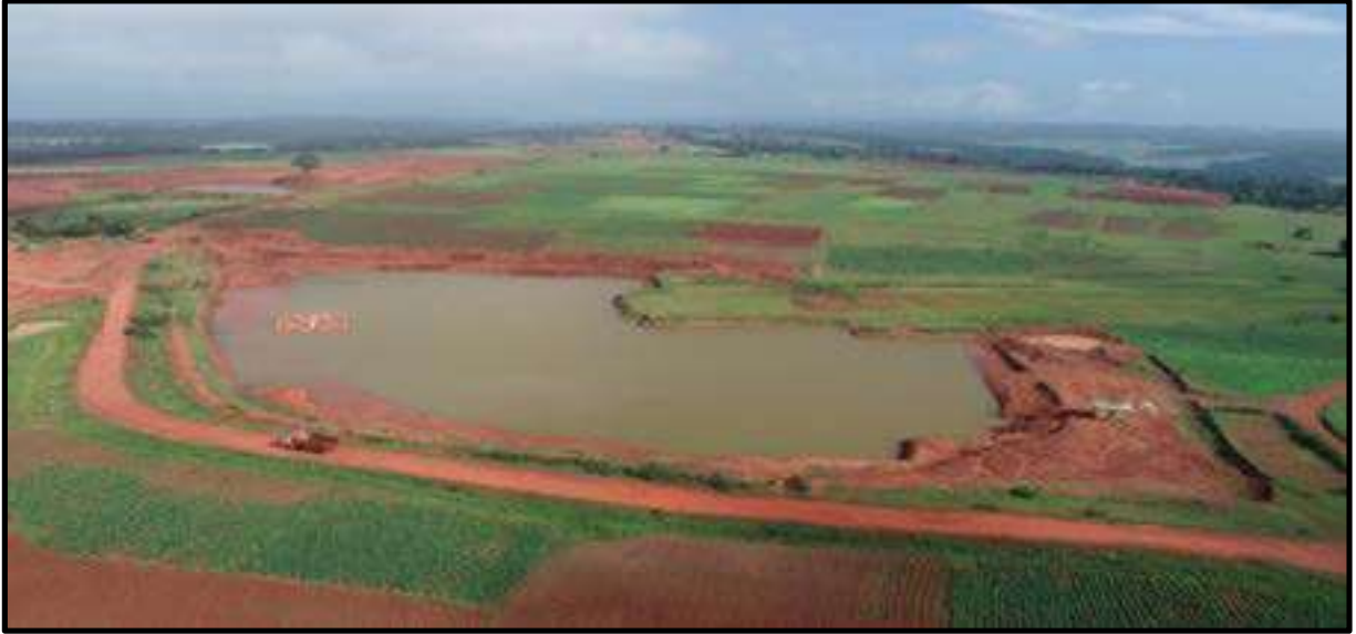
(Rainwater harvesting pond)
