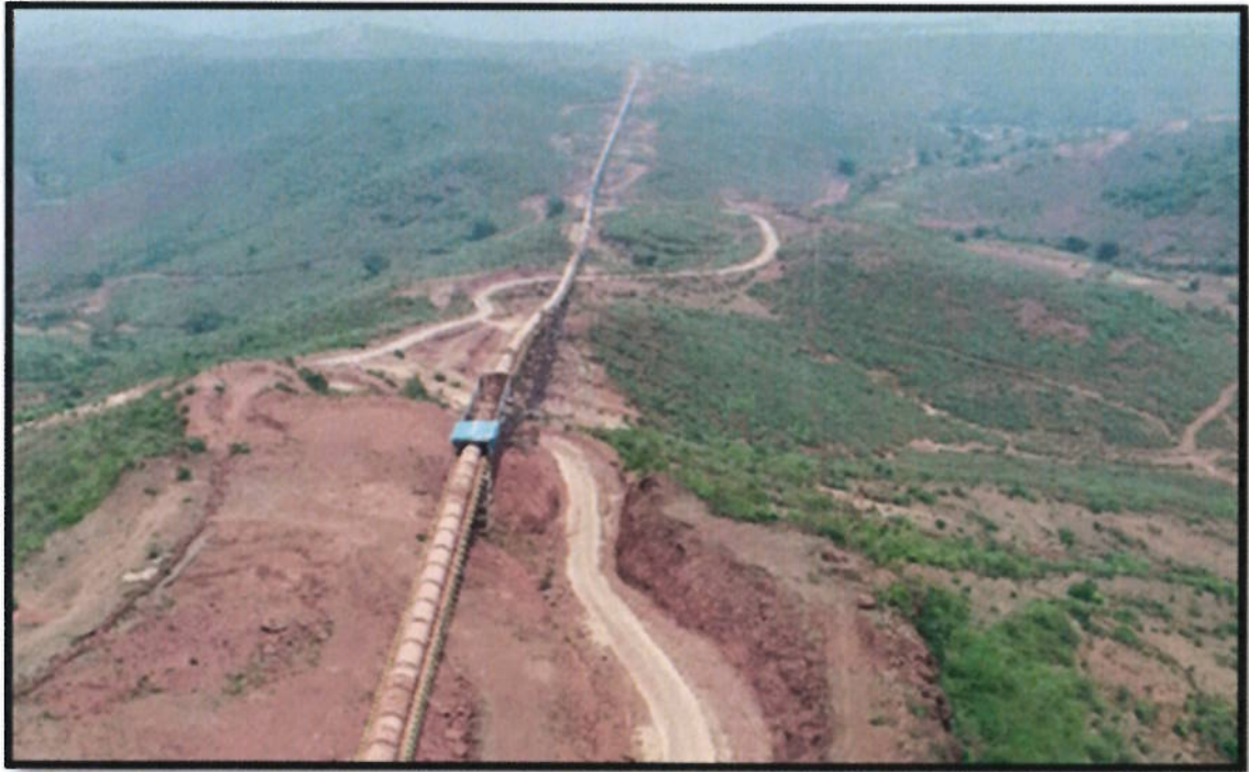
Photo -11 : Showing conveyor with covered metal hood for transportation
