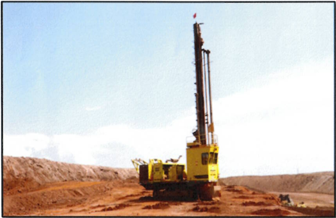
Photo -9 : Showing drilling operation with dust extractor system
