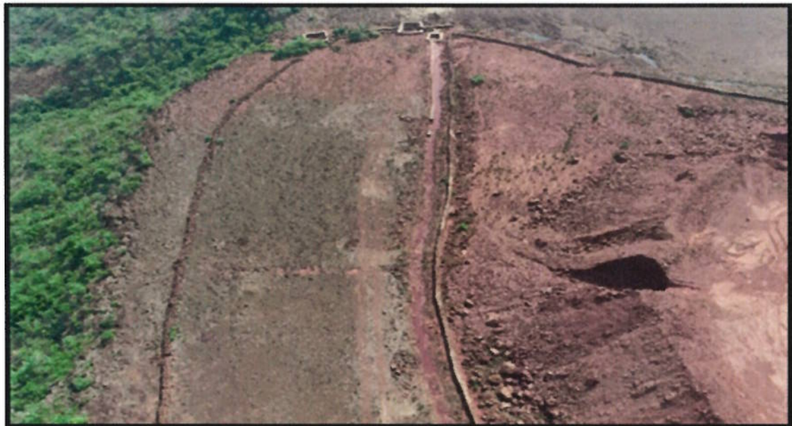
Photo -2 : Showing Retaining wall & garland drain around dump slope
