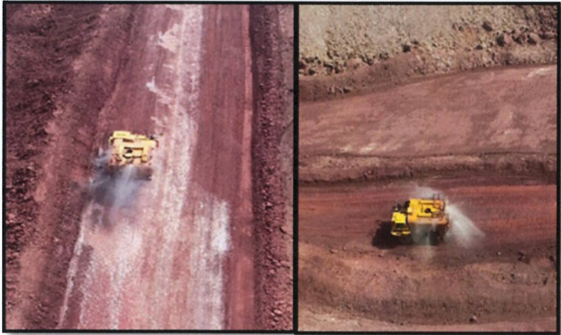
Photo -7 : Showing Mobile water sprinklers in operation
