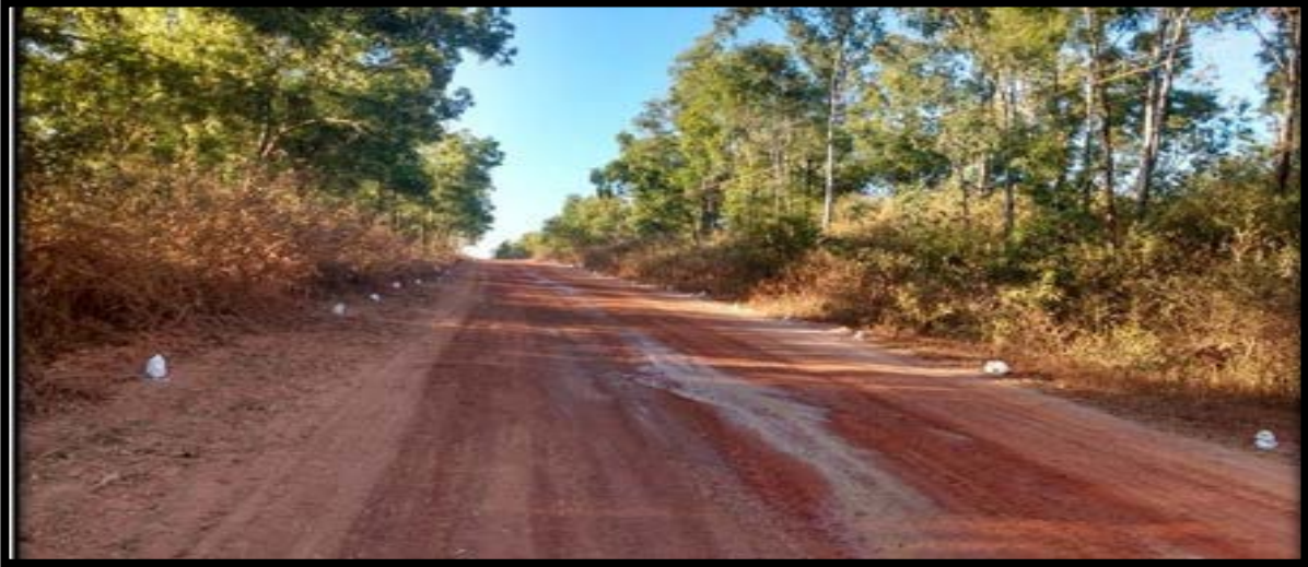
Green Belt Development along Road side
