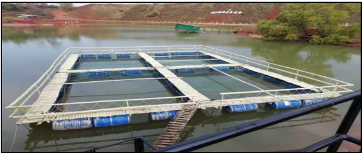
Rainwater Harvesting pond at Bagru
