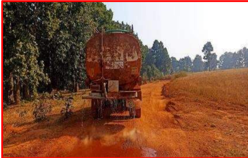
Water Sprinkling through tanker
