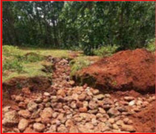
Catchment drain & Siltation Pond
