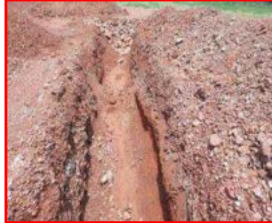
Catchment drain & Siltation Pond
