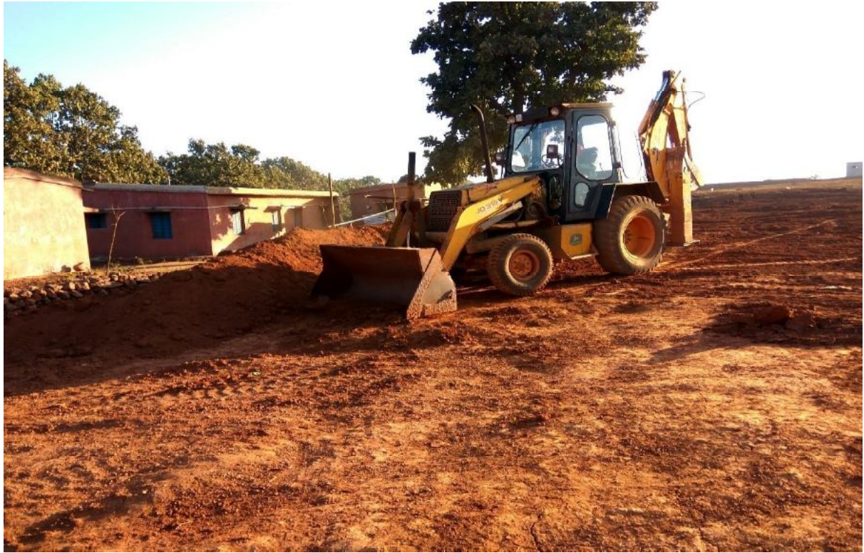
Reclamation process is going on over mined out area
