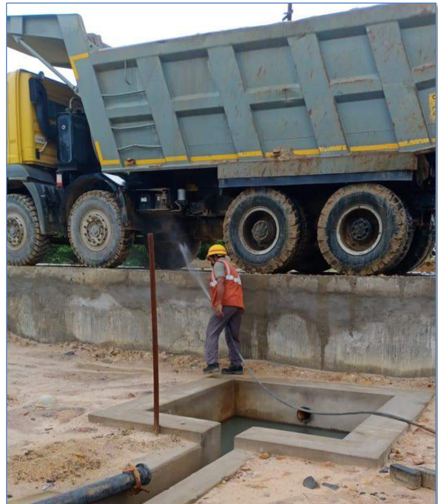
Dumper/HEMM Washing Bay at Bankheta – GP IV/4 Coal Mine
