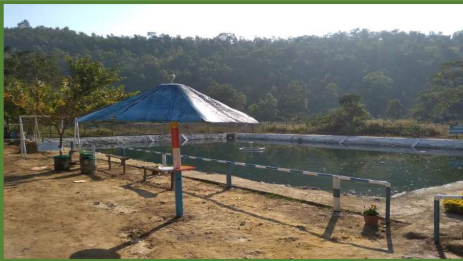
SETTLING POND NO – 3
