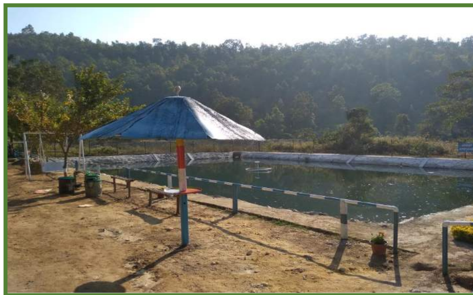
SETTLING POND NO – 3
