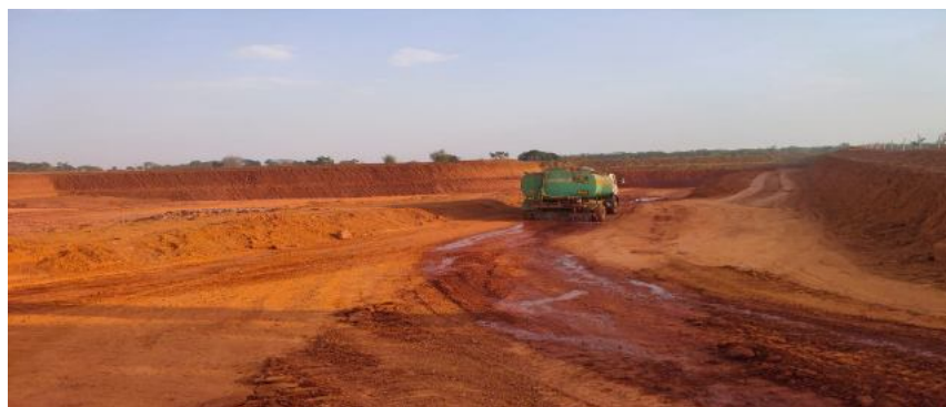
WATER SPRINKLING ON HAUL ROAD
