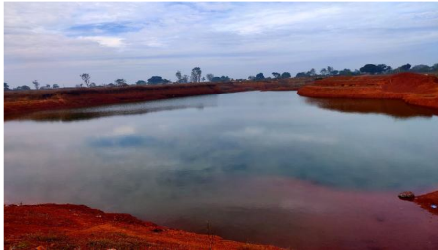
RAINWATER HARVESTING POND
