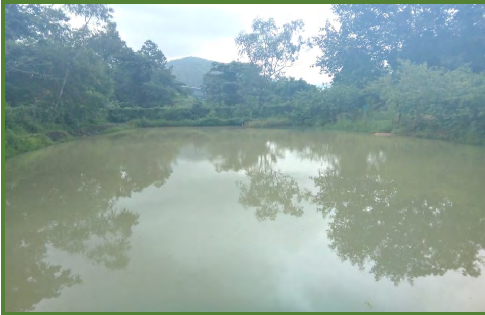
SETTLING POND NO – 1
