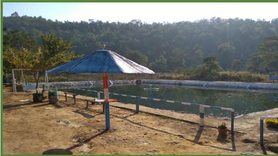
SETTLING POND NO – 3
