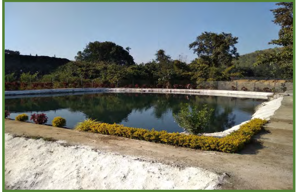
SETTLING POND NO – 2
