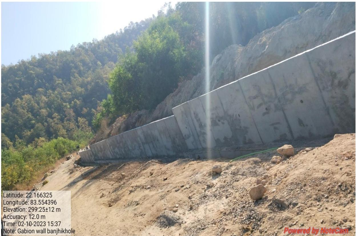
Total 105 m gabion/retaining wall constructed in this Quarter (Nov'22 – Jan'23) at Patch "C"
