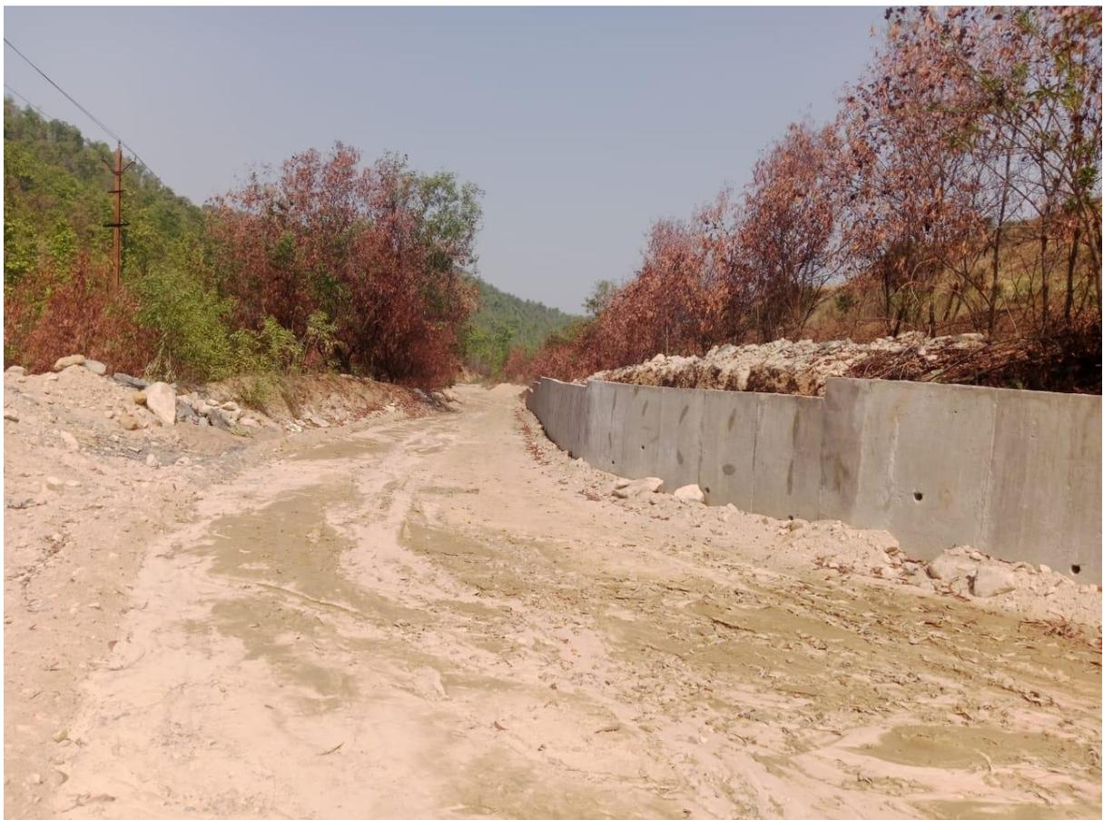
Total 55 m gabion/retaining wall constructed in this Quarter (Feb'23 – Apr'23) at Patch "C"
