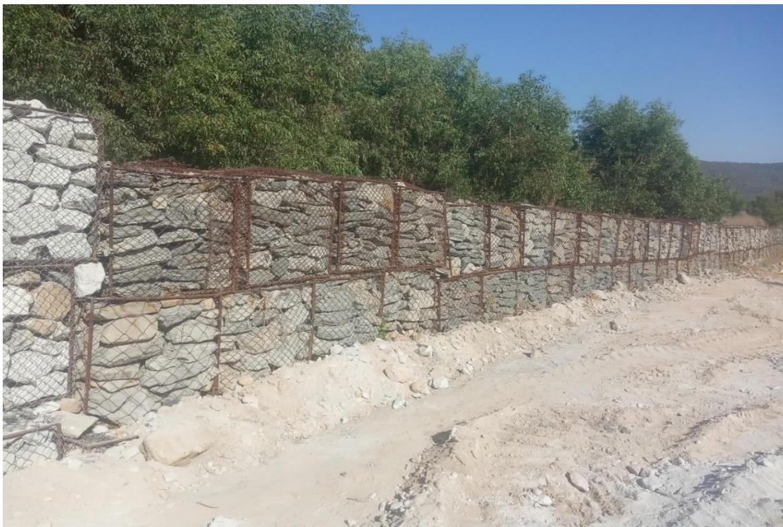
In the 1st Phase HIL has constructed approx. 55 mtr. long gabion/retaining wall at the toe of permanent dump slope near Patch "C" in Banjikhhol, GP IV/4 Coal Mines.
