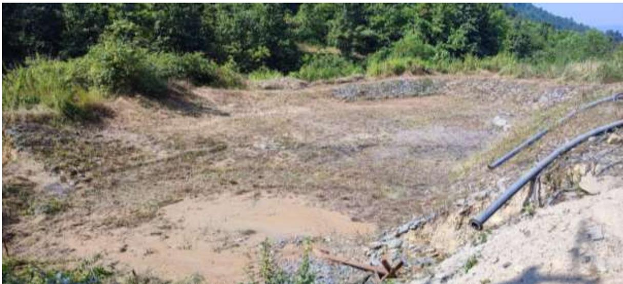
HIL constructed an additional settling pond of size 30m X 10m X 1.5m (01Nos) to collect whole mine seepage water generated during the mining activities from Patch “C” specially in the rainy season for proper settling of mine seepage water before discharge
