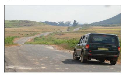
Laxmipur Jn. To Sorispadar (23.8 Km) under construction, For transportation of heavy project materials to site (15 kms Black Topping completed
