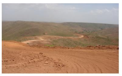
Mines Road: road work under progress to make it motorable (21 Km)
