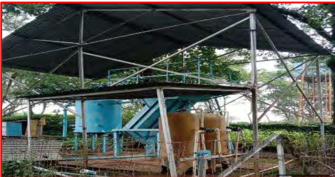
Sewage Treatment Plant
