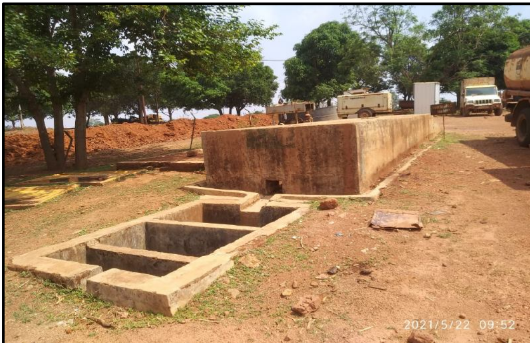
(Washing Ramp and Oil and grease trap)
