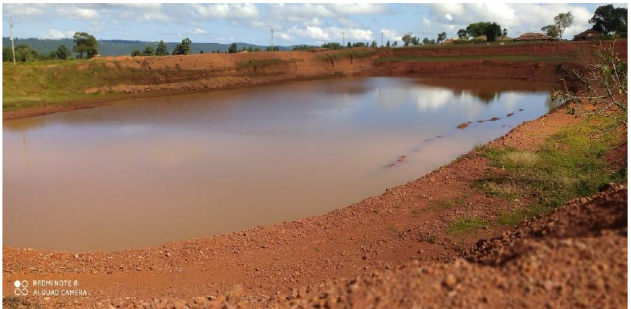
Pic: Shows Southern view of Water Pond (Rain water Harvesting Pond) at Kujam-I Bauxite Mines.
