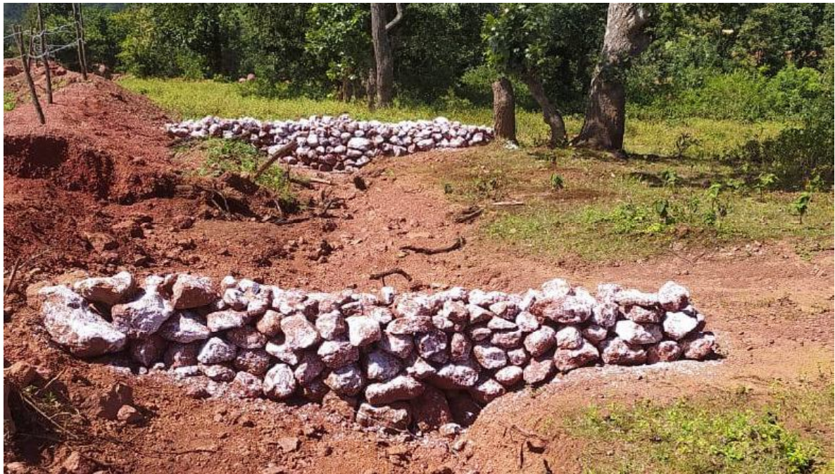
Retaining wall to prevent solid wash-off
