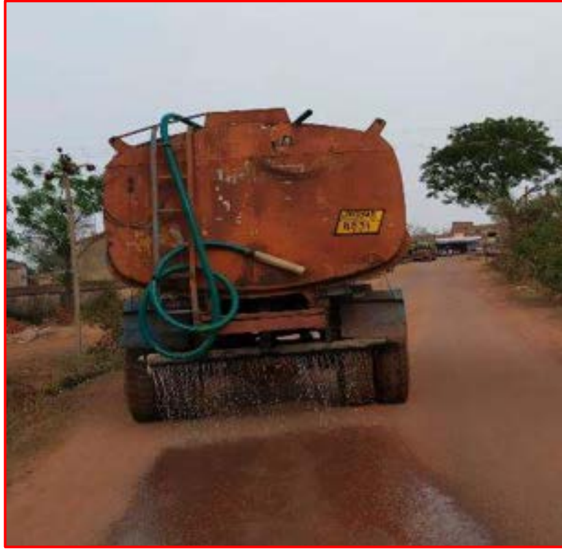
Water sprinkling through tanker
