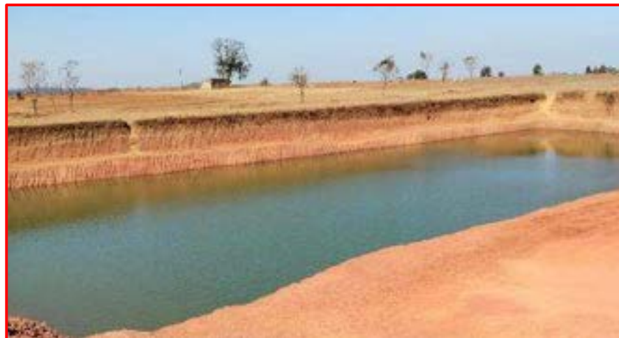
Rainwater Harvesting Pond
