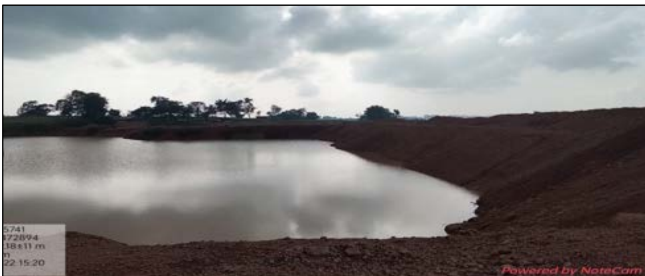
Rainwater Harvesting Pond
