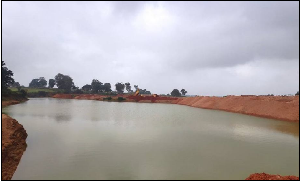
(Rainwater harvesting pond)
