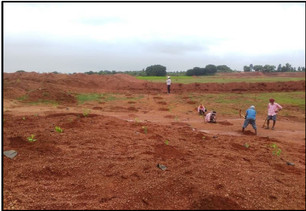
(Plantation over reclaimed area)
