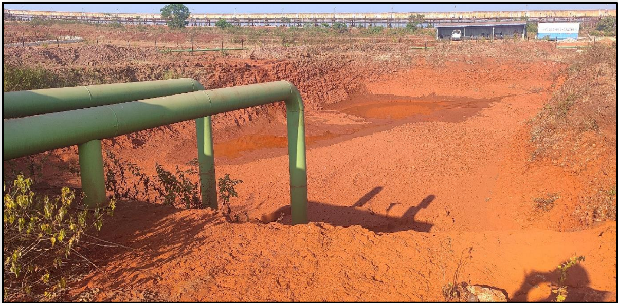
Settling Pond-1 Near Mines Entrance
