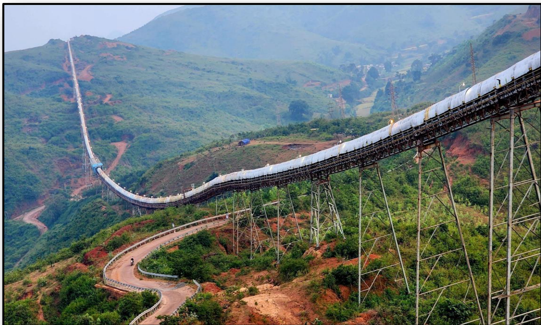
PHOTO 13: Showing Covered Long-Distance Conveyor (LDC)
