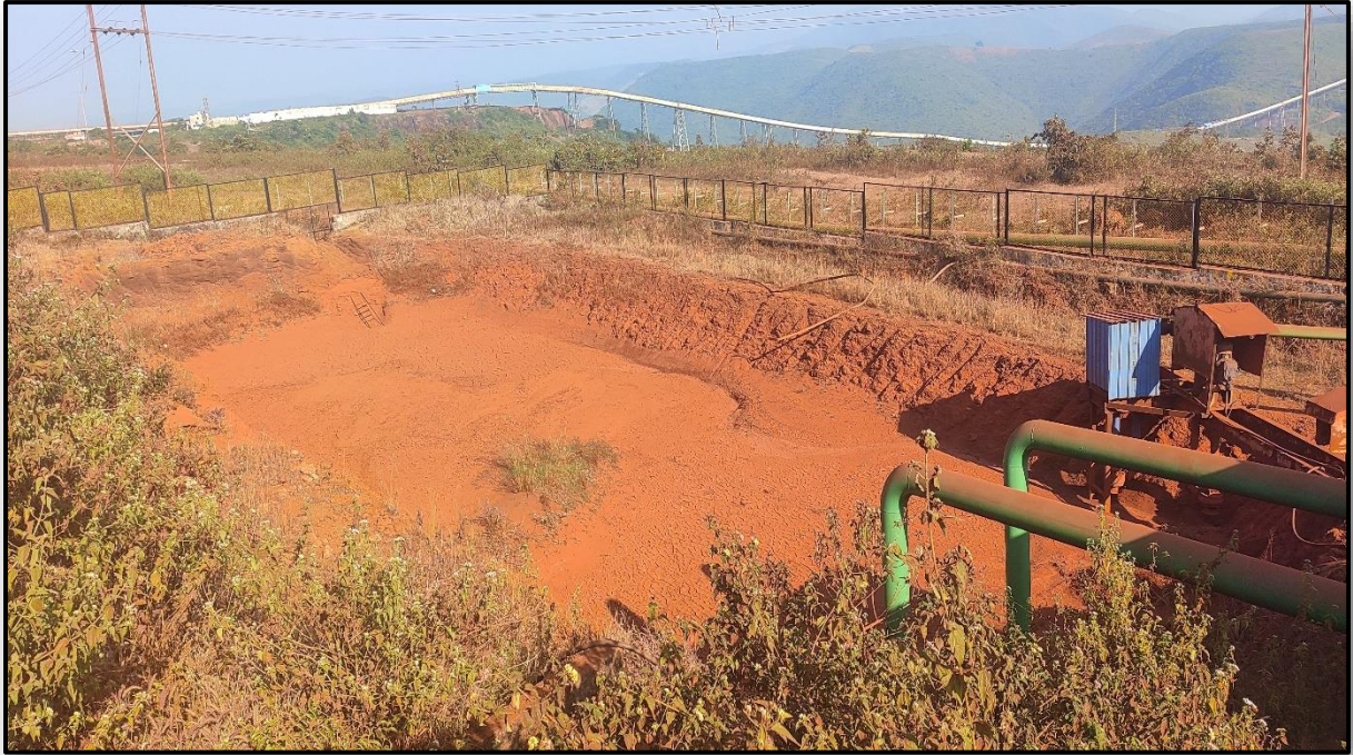
Settling Pit Near Crusher House
