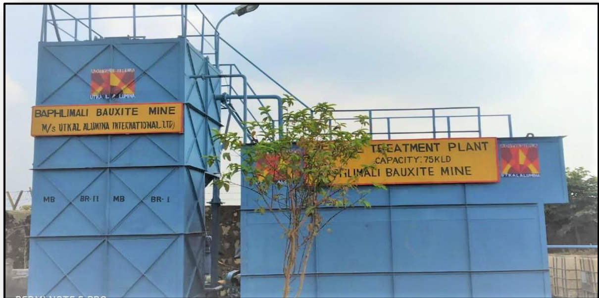
PHOTO 15: Showing 75 KLD Sewage Treatment Plant(STP)
