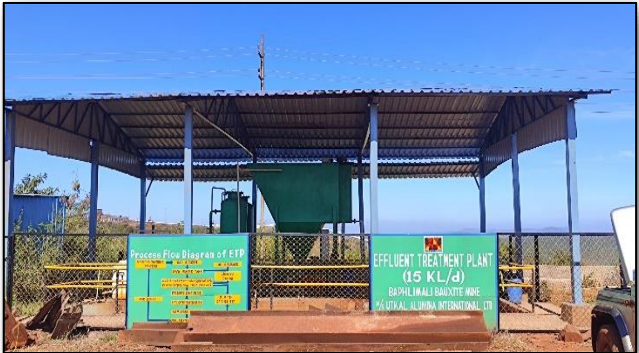
PHOTO 16: Showing 15 KLD Effluent Treatment Plant(ETP)
