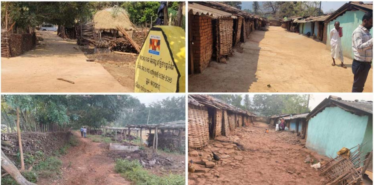
Before and after photos of connecting road of Kadapadar village
