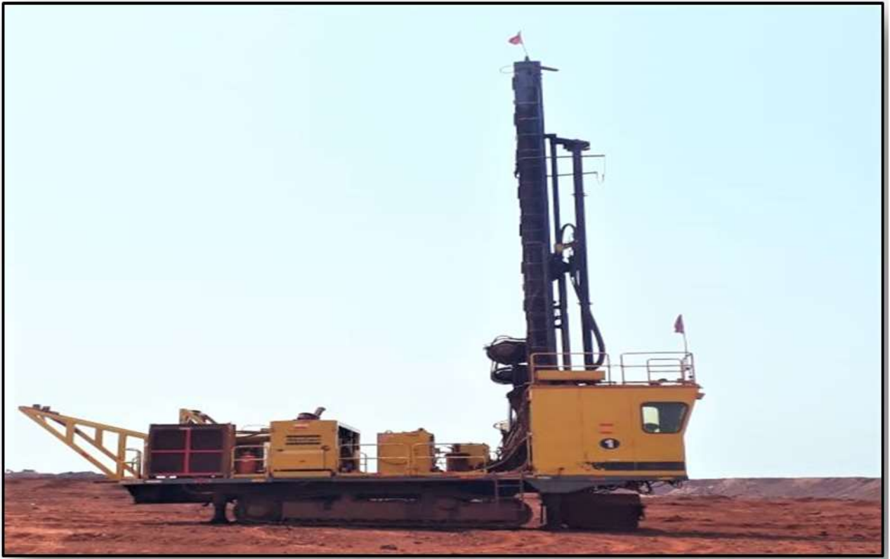
PHOTO 12: Showing drilling machine with dust Extractor.
