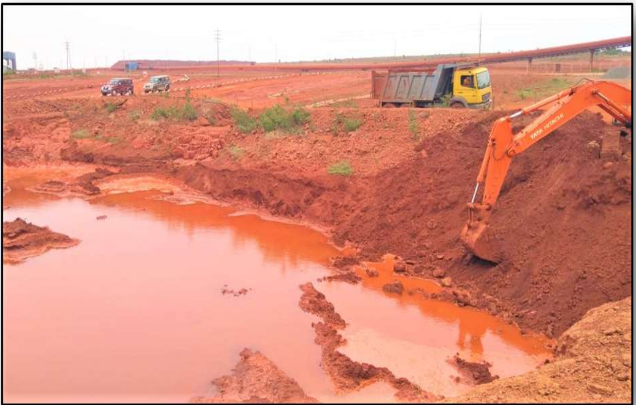
PHOTO 4: Showing Settling Pond Desilting
