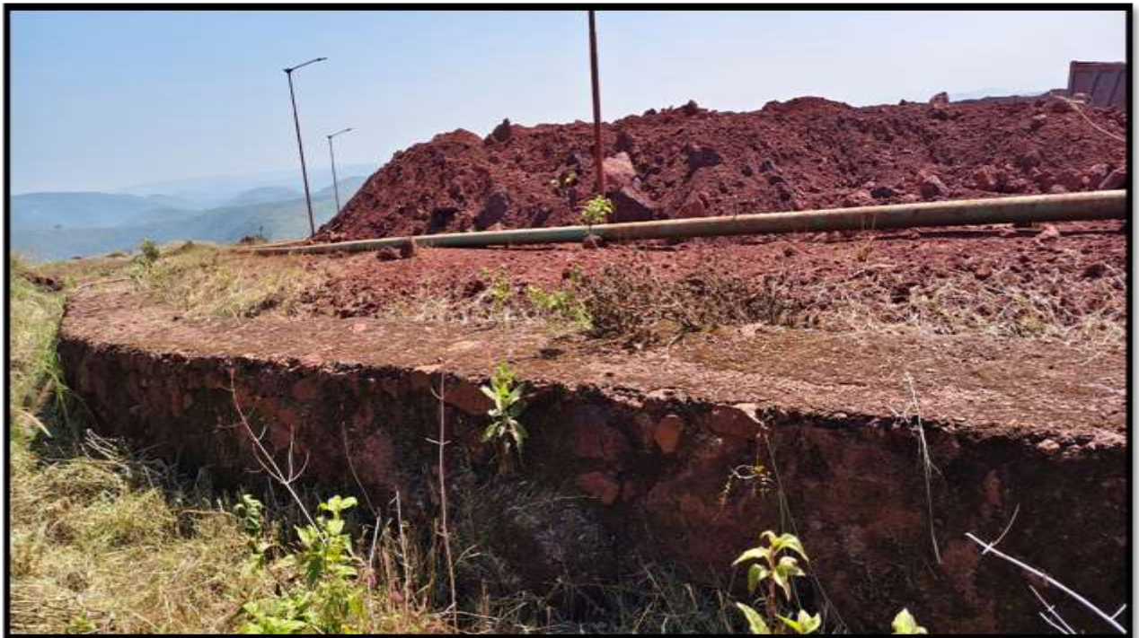
PHOTO 2: Showing garland drain along the storage stake yard.
