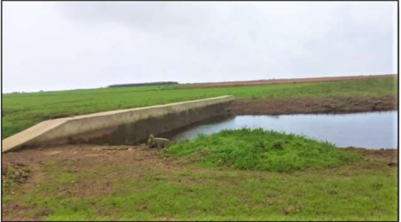
PHOTO 1: Showing Check dam
