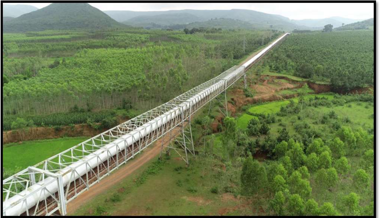
PHOTO 14: Showing Covered Long-Distance Conveyor (LDC)
