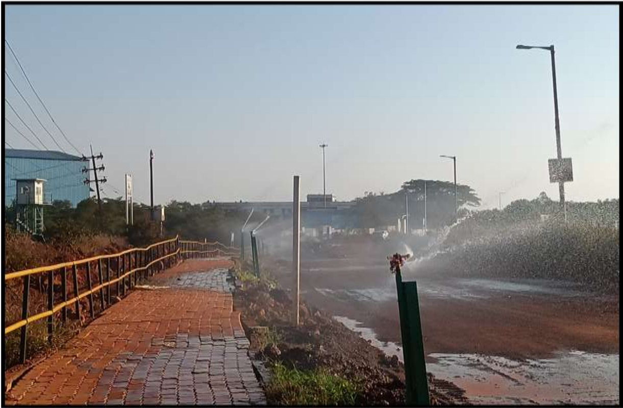
PHOTO 9: Showing Fixed Sprinklers
