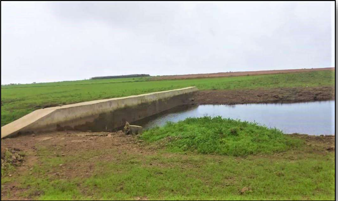
PHOTO 1: Showing Check dam
