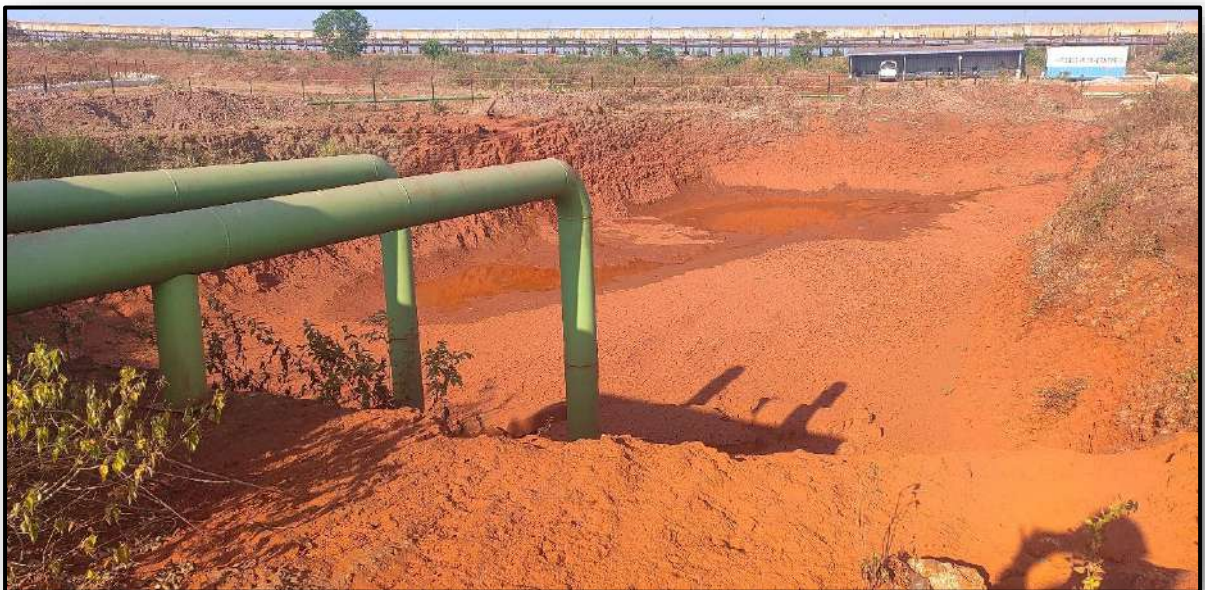
Settling Pond-1 Near Mines Entrance
