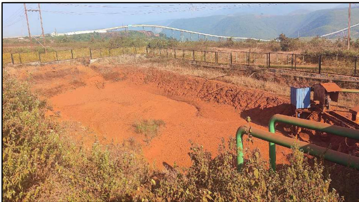
Settling Pit Near Crusher House
