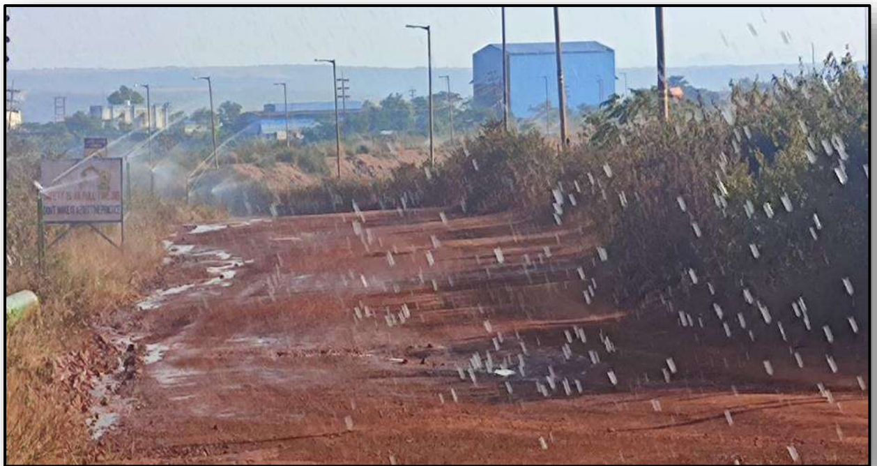
PHOTO 9: Showing Fixed Sprinklers
