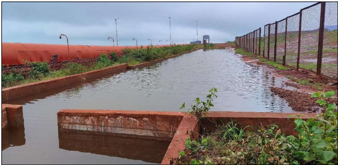
PHOTO 11: Surface Rainwater Harvesting Structure.
