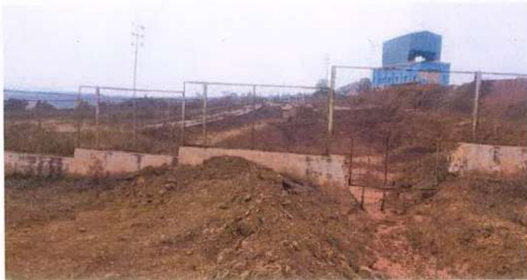
Figure 10: Fencing around the settling pit
