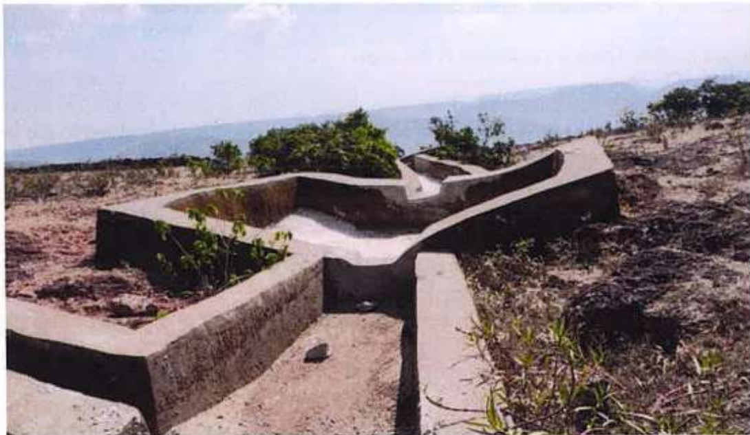
Figure 7: Renovated settling pits
