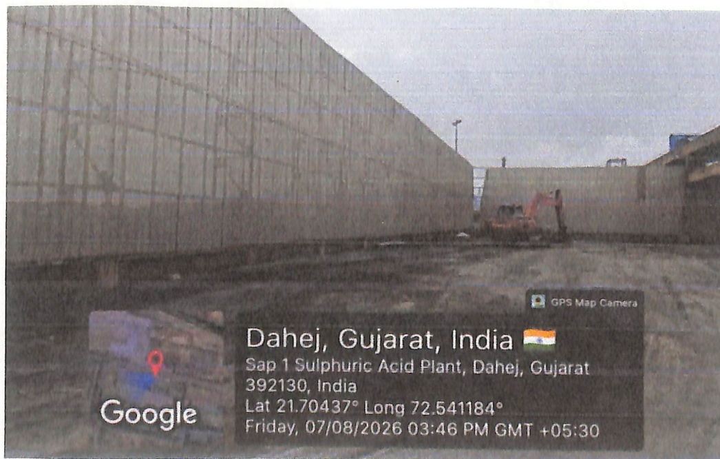
Figure 5: Temporary/emergency ash storage facility
