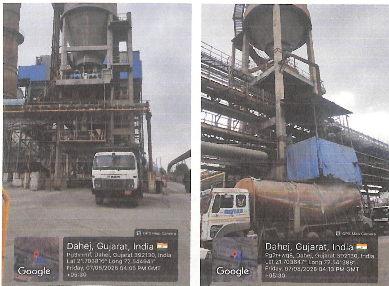
Figure 6: Dry fly ash silo at captive power plant, Hindalco Industries Ltd. (Unit: Birla Copper, Dahej), Gujarat
