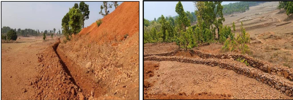
Photographs of garland drains and parapet wall
