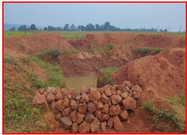
Retaining wall and siltation pit to prevent solid
