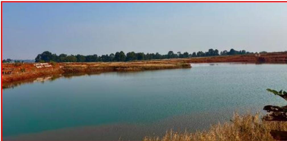
Rainwater harvesting structure
