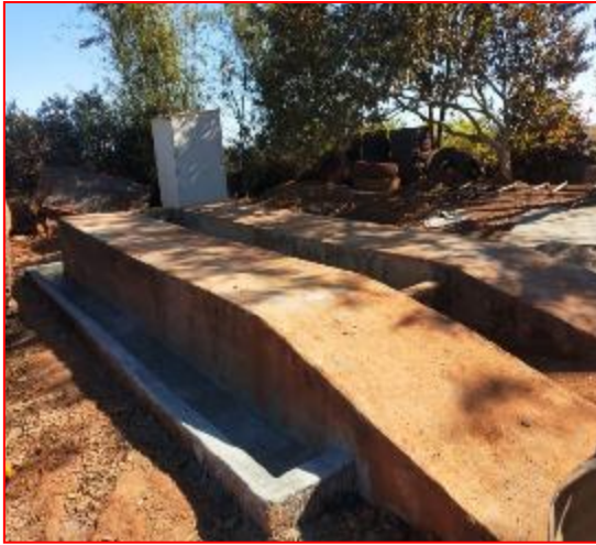
Oil and Grease Trap at Mines
