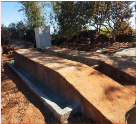
Oil and Grease Trap at Mines
