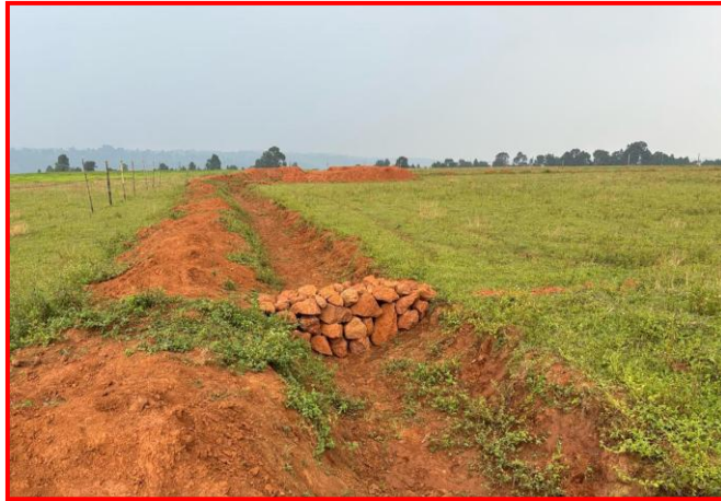
Retaining wall and siltation pit to prevent solid
