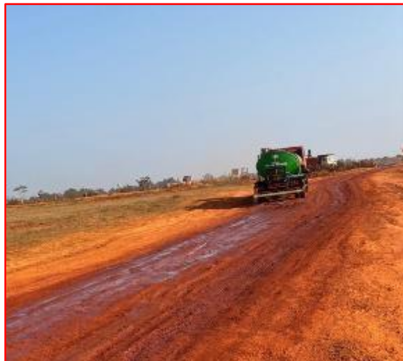
Mobile water tanker for dust suppression
