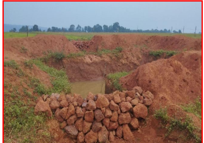
Retaining wall and siltation pit to prevent solid
