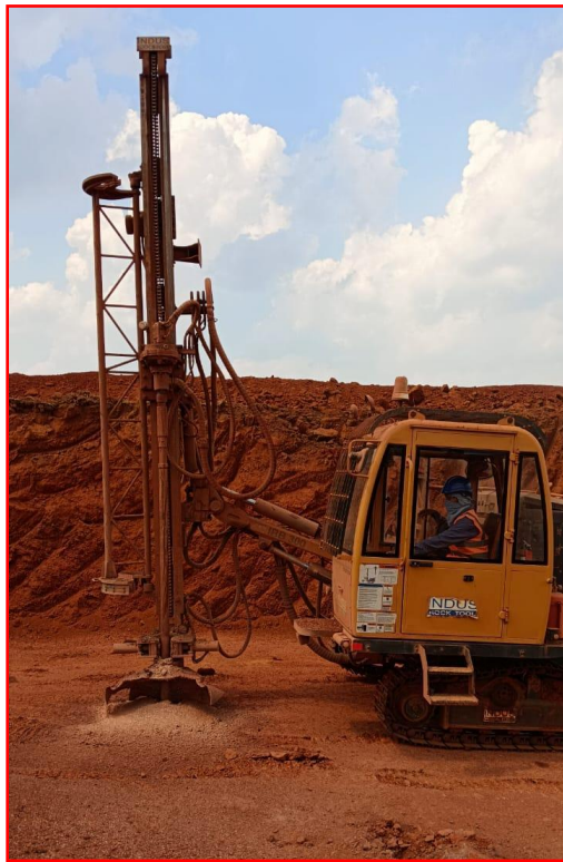
Wet drilling is in practice.
