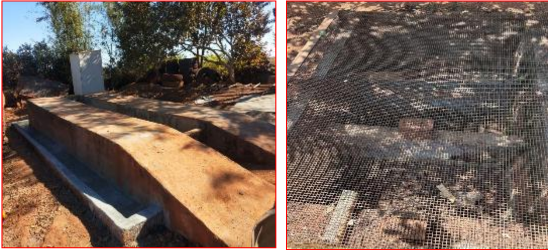
Oil and Grease Trap at Mines
