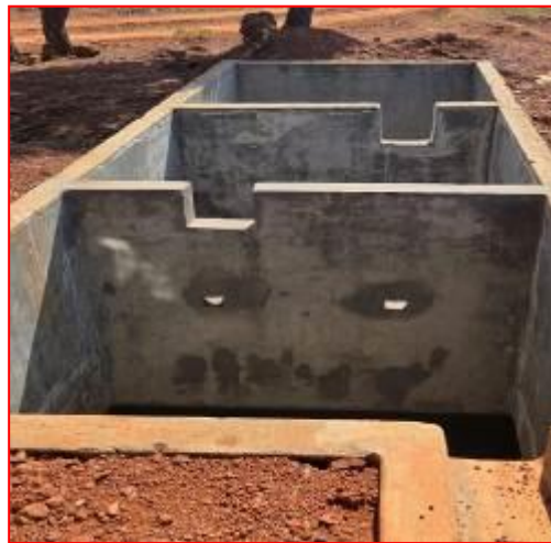
Washing Ramp with Oil and Grease trap
