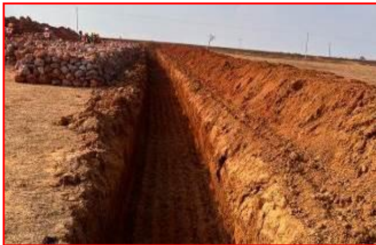
Garland drains around Mine Pit
