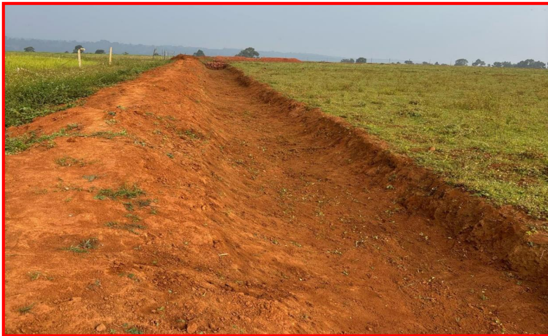
Garland drains around Mine pit.
