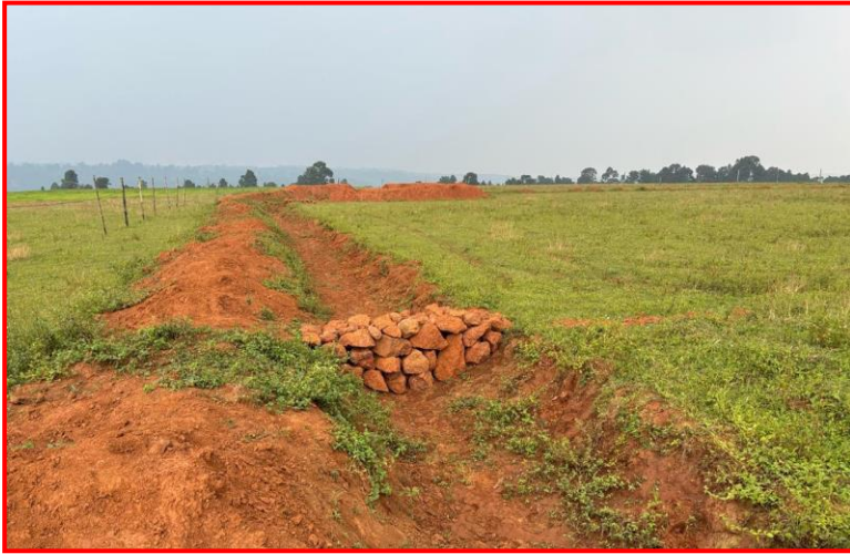
Retaining wall and siltation pit to prevent solid wash-off.
