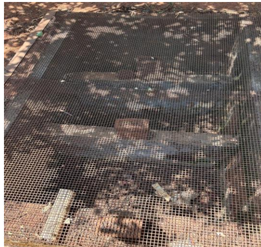
Oil and Grease Trap at Mines
