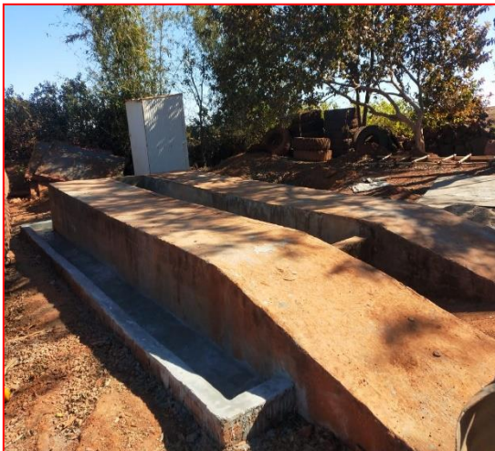
Oil and Grease Trap at Mines
