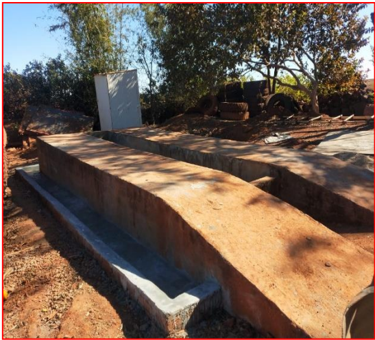
Oil and Grease Trap at Mines
