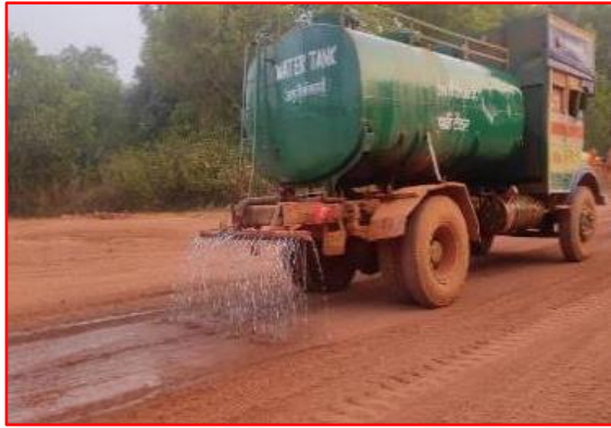
Dust suppression through water tanker
