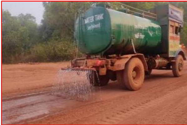
Dust suppression through water tanker
