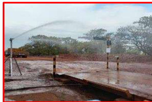
Fixed Type Water Sprinkler
