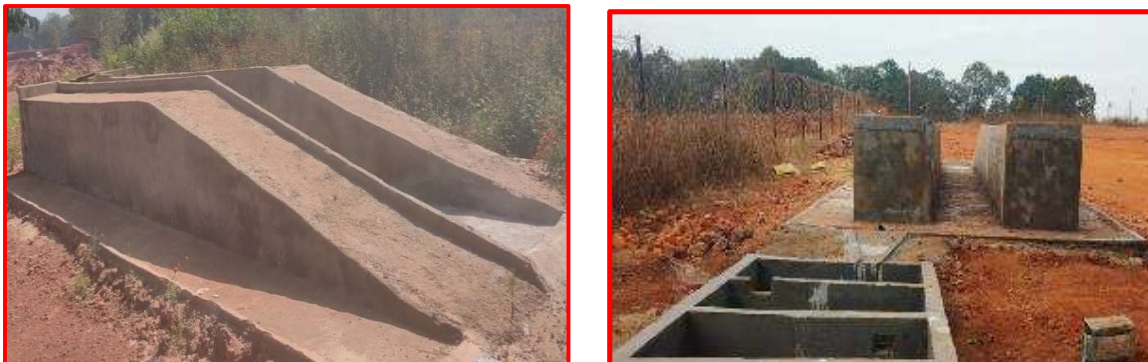
Washing Ramp with Oil and Grease Trap System
