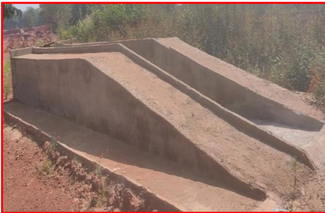
Washing Ramp with Oil and Grease Trap System
