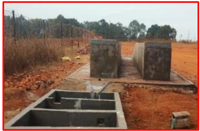
Washing Ramp with Oil and Grease Trap System
