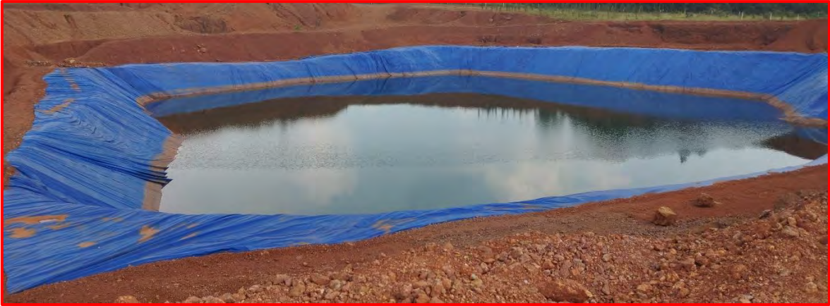
Rainwater Harvesting Pond
