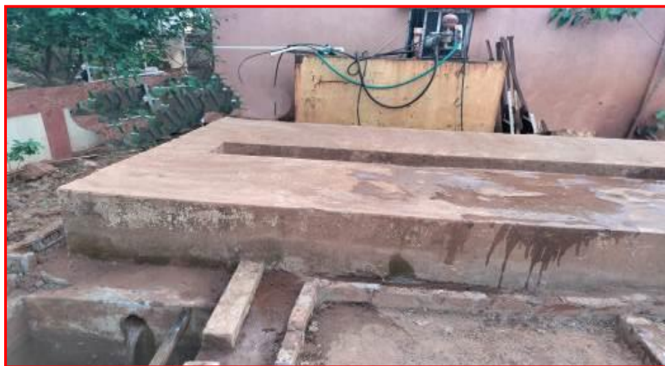
Washing Ramp with Oil and Grease trap
