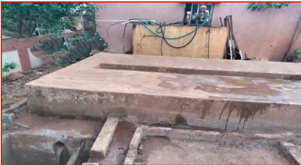
Washing Ramp with Oil and Grease trap
