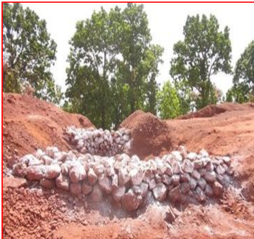
Catch drain Near mine pit.
