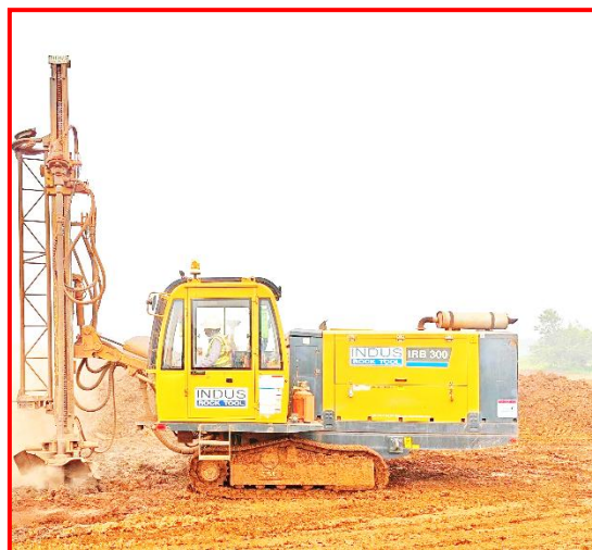
Wet drilling is being carried out.
