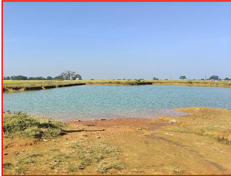
Rainwater Harvesting Pond.
