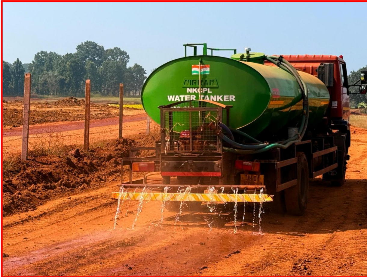
Water Tanker for dust suppression
