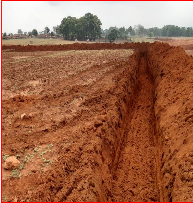
Garland drain around mine pit.
