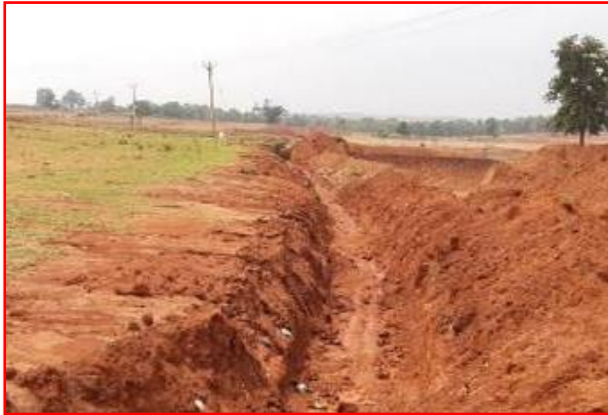
Garland drain around mine pit.
