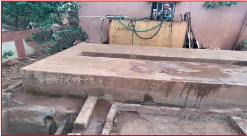
Washing Ramp with Oil and Grease trap
