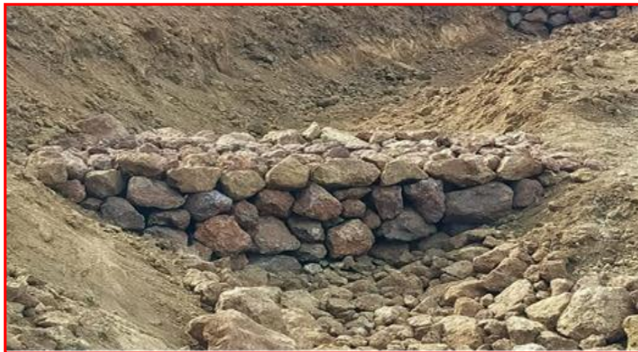
Catch drain Near mine pit.
