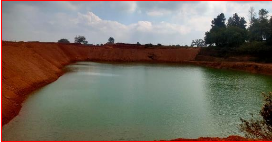
Rainwater Harvesting Pond
