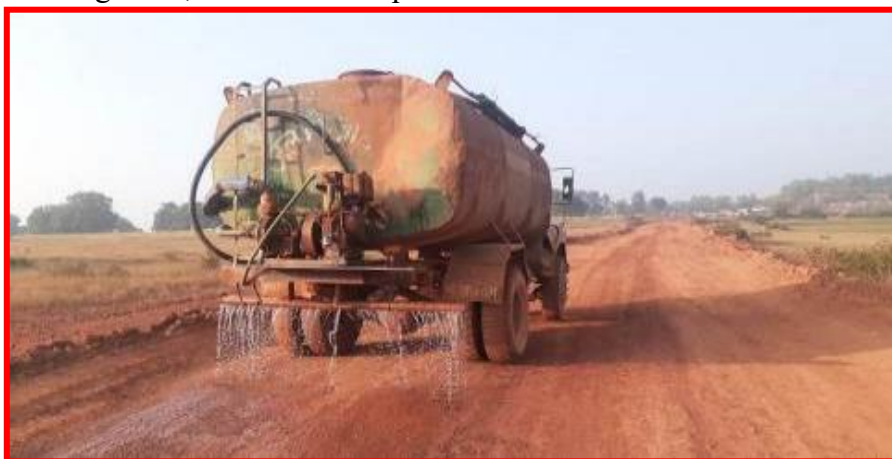
Water sprinkling through Tanker
