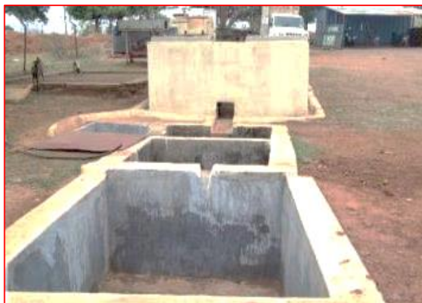
Washing Ramp and Oil and Grease Trap
