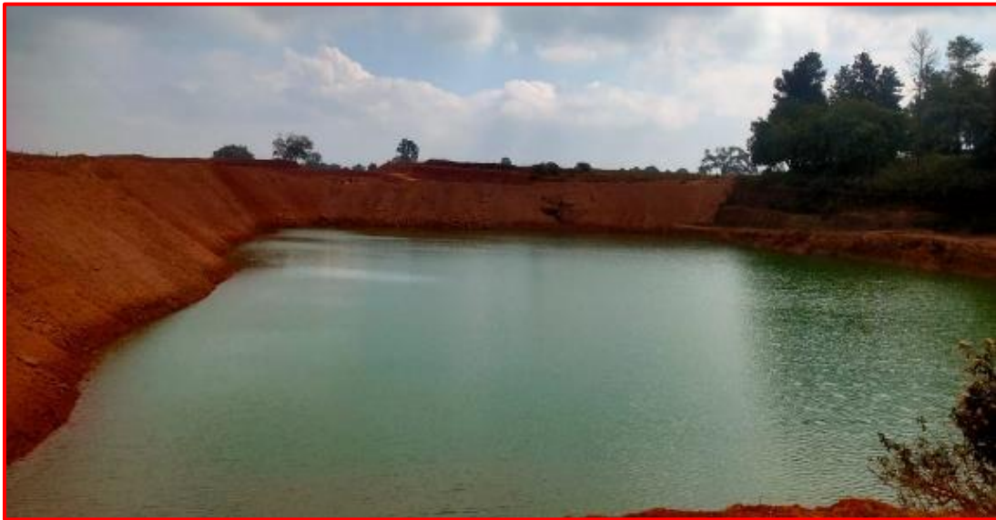
Rainwater Harvesting Pond
