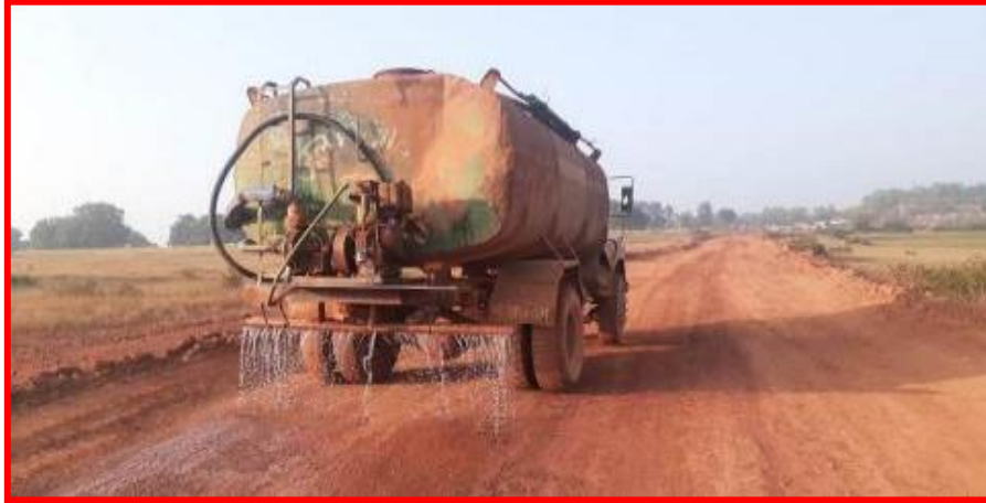
Water sprinkling through Tanker
