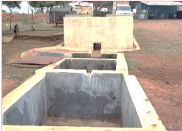
Washing Ramp and Oil and Grease Trap
