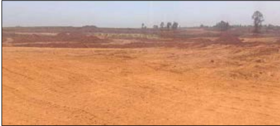
Topsoil Spreading for Backfilling
