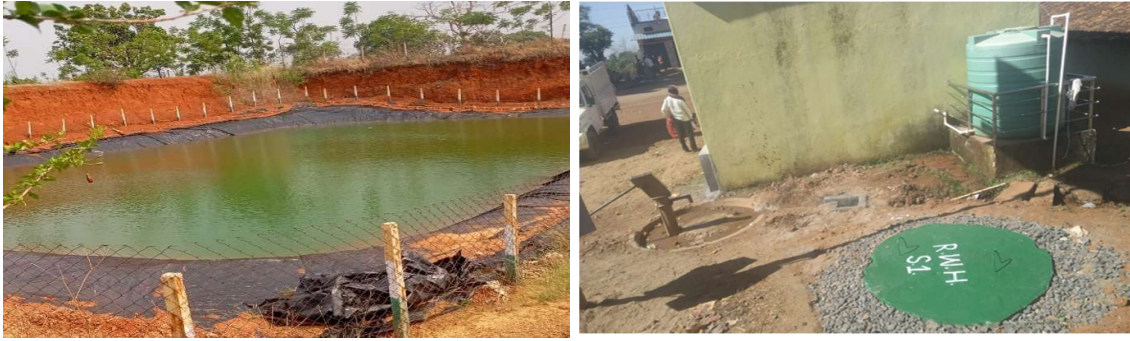
RWH Pond & Well Structure
