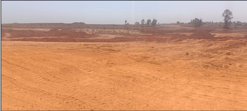
Topsoil Spreading for Backfilling
