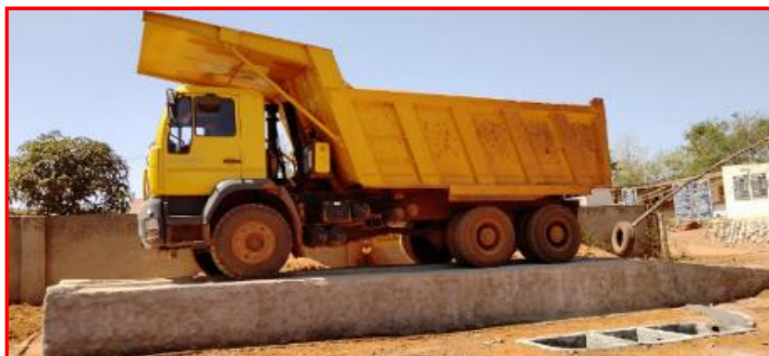
Washing ramp with Oil and Grease Trap
