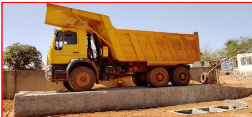
Washing ramp with Oil and Grease Trap
