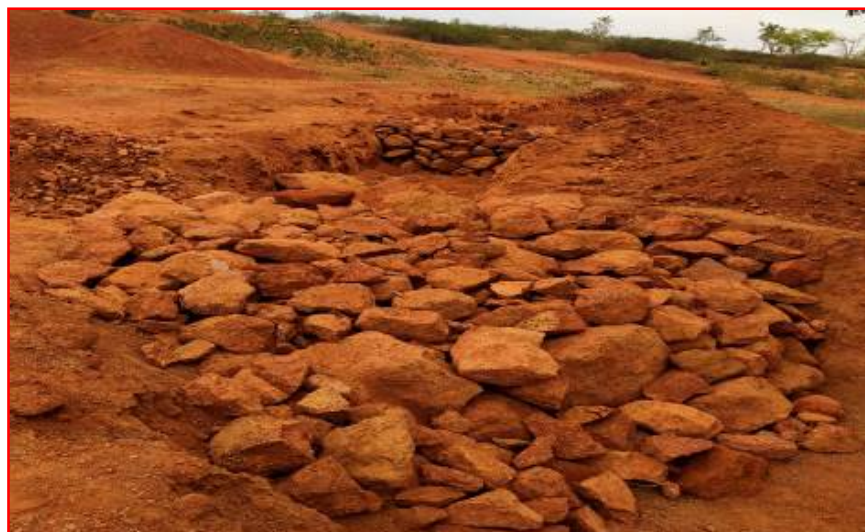
Check drain and Siltation pit around mine pit to prevent runoff.
