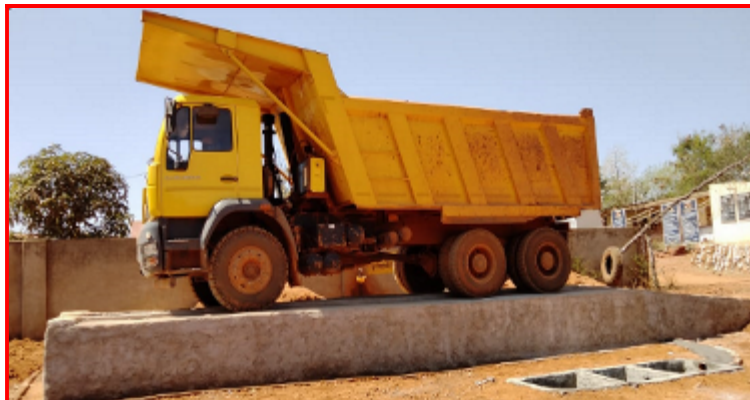
Washing Ramp with Oil and Grease Trap
