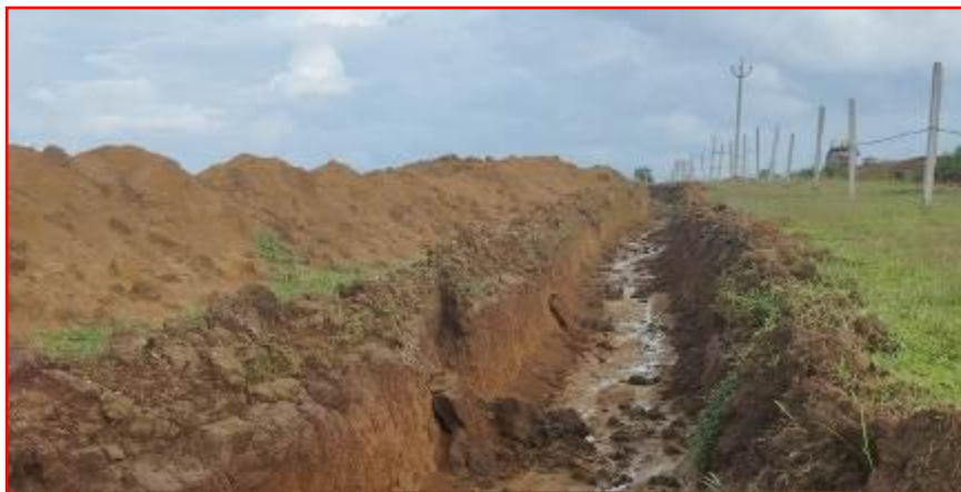
Garland drains around mine pit to prevent runoff.
