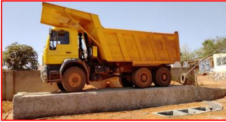
Washing Ramp with Oil and Grease Trap
