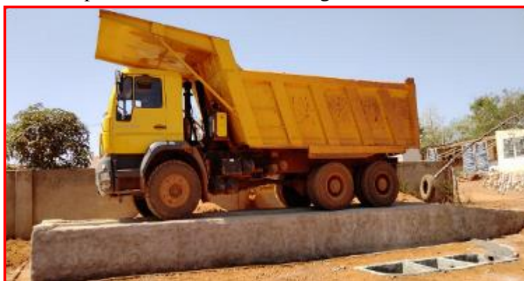
Washing Ramp with Oil and Grease Trap
