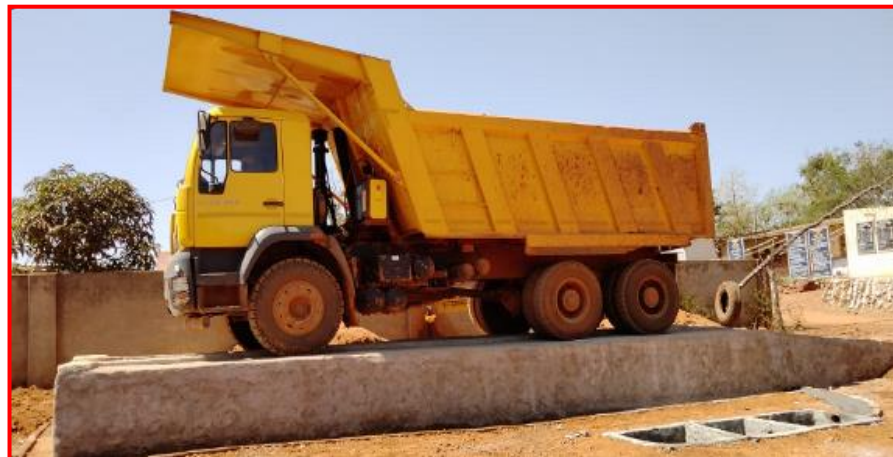
Washing Ramp with Oil and Grease Trap
